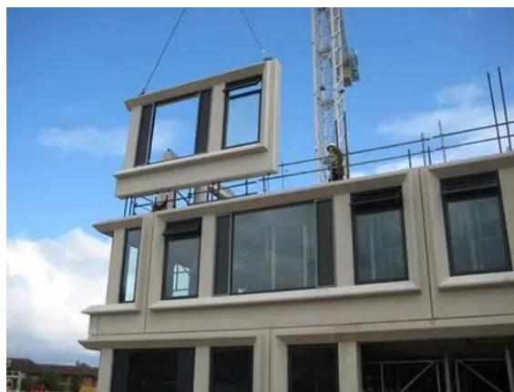
Figure 1: Prefabricated building construction.
